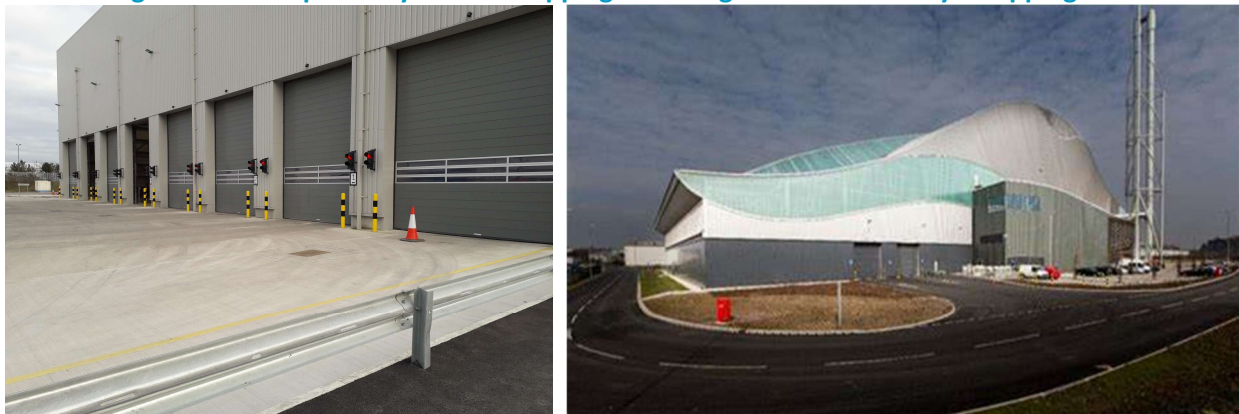
Figure 4-1 multiple entry doors to tipping hall & Figure 4.2 Dual entry to tipping hall
